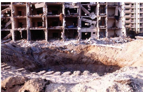
Figure 5-1: Khobar Towers Dhahran, Saudi Arabia, 1996 (Source: DOD Photo)
