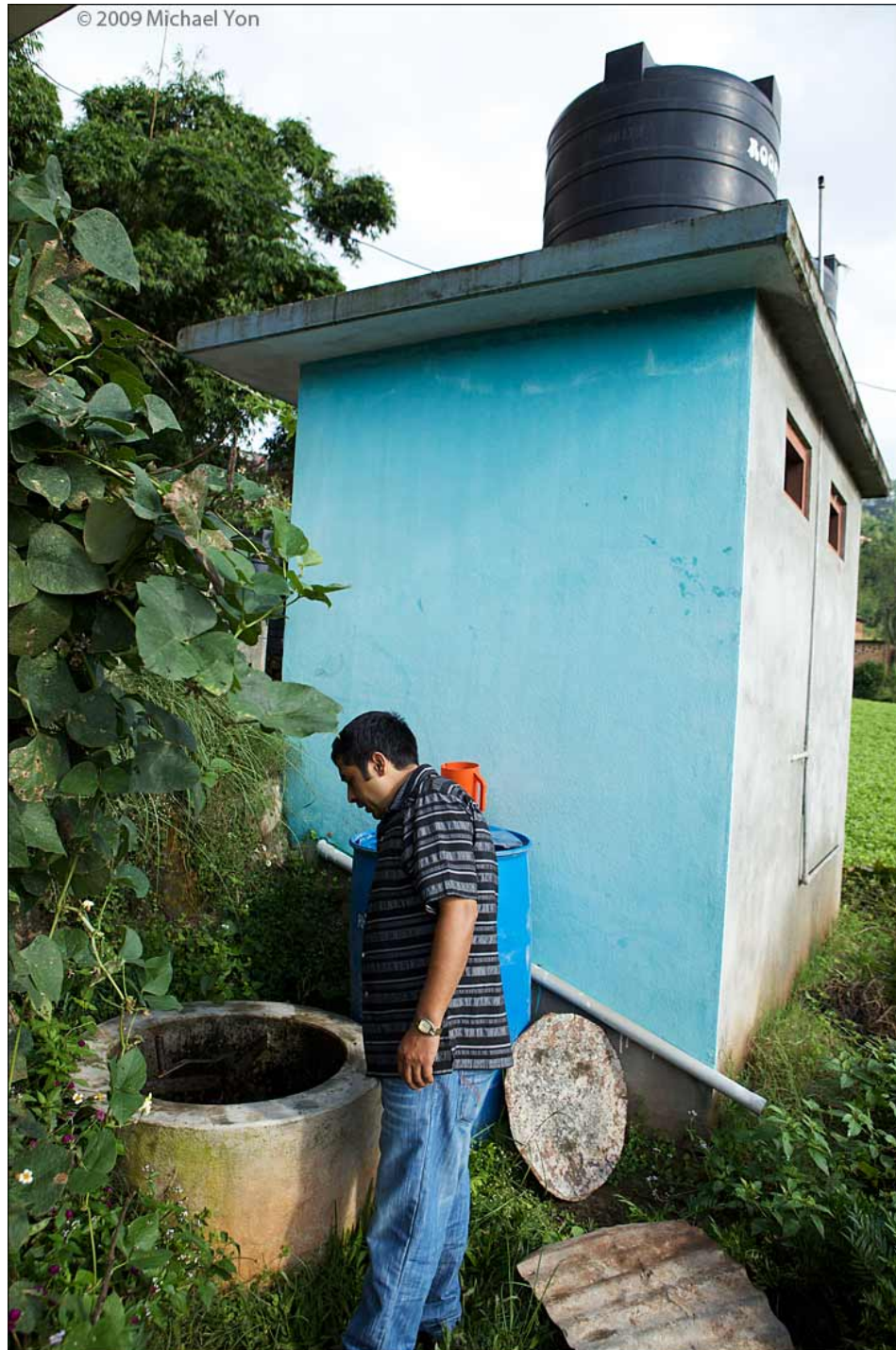
Nepalese Gobar Gas: this installation begins at the blue outhouse. Human waste feeds to the underground “digester.”
