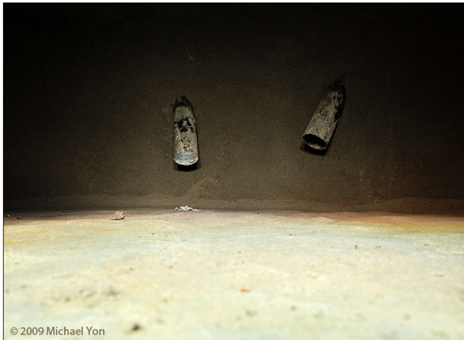
Both pipes meet underground in the digester. Normally this place is filled with tons of excrement. This digester was under construction. One pipe stems from the mixer, the other from the outhouse.
